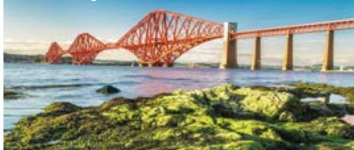
Firth of Forth bridge
